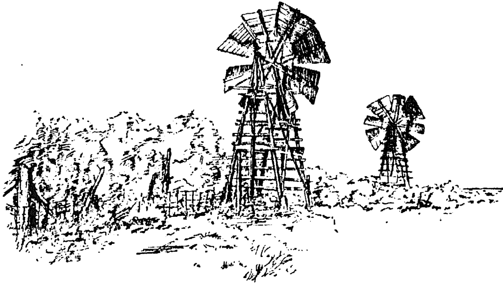
FIG. 49. Twin Battle-ax windmills on the thousand-acre farm of Mr. J. S. Peckham, near Gothenburg, Nebraska. Towers are made of four-by-fours, cross-braces of two-by-fours; stand twenty feet high. Diameter of wheel sixteen feet; fans five and one-half feet long, five feet wide at the top tapering to two and one-half to three feet at the bottom. Used in irrigating a fifteen-acre orchard. Capacity of each will average nearly one thousand gallons an hour in a fifteen mile wind. Cost $25 each.
