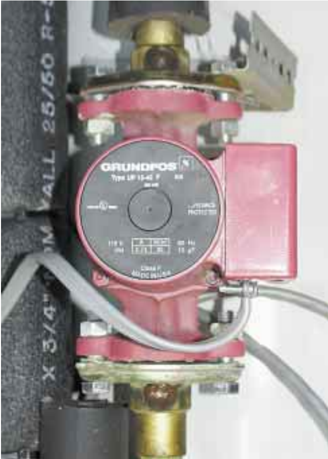
The Grundfos UP 15-42 F is a typical AC circulating pump for closed loop systems.
