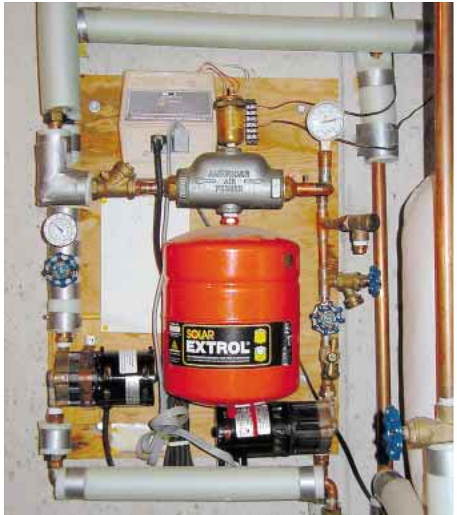
A closed loop module groups the major components on one board. This homebrew model by the author has functioned without fail since 1982.
