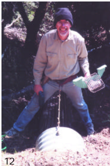
12. With my old tower safety belt secured to a bolt I had added to the northern culvert, I worked hands-free adding the culvert dam.
