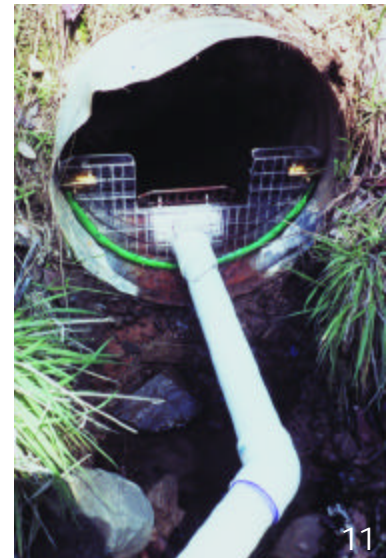
11. PVC pipe attached to the culvert dam is not glued so that it may be easily removed.
