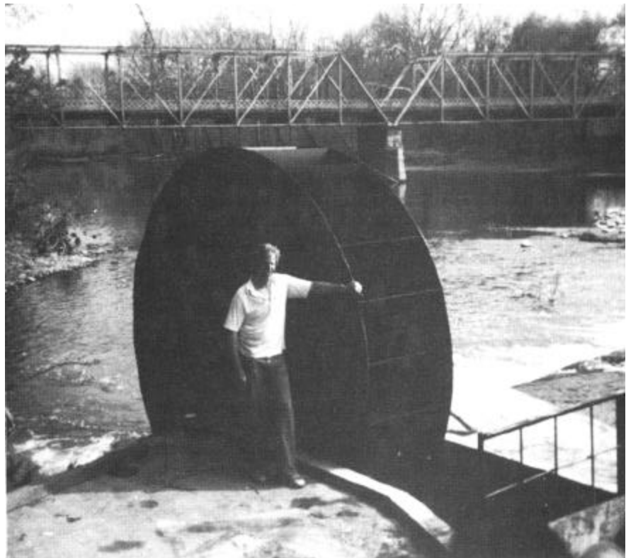
A FITX Waterwheel Company all-welded steel undershot wheel.
