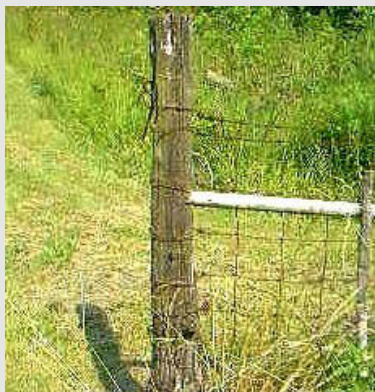
An Osage Orange Corner post of about 8 inches in diameter that has been in the ground for over 20 years.
