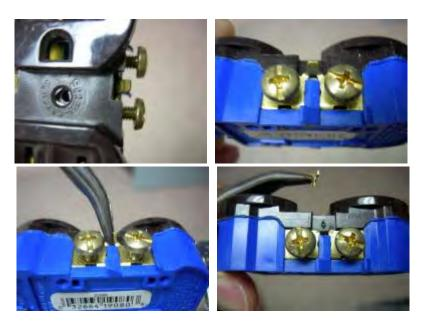
The first two graphics show the metal strip or tab. The third and fourth graphics show how the tab is easily removed with a set of needlenose pliers. Once the tab is removed, the upper and lower outlet plugs are independent so one can be, for example, controlled by a wall switch while the other is always on. If you have a split outlet, follow the same 3-way switch troubleshooting as with a light fixture EXCEPT you will need to determine which outlet is always on.
