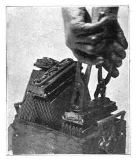
Fig. 165. Lifting Elements Out of Jars, and Resting on Edge of Case to Drain. Willard Type S Battery
