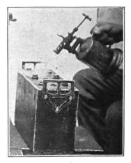
Fig. 103. Heating Compound with Torch
