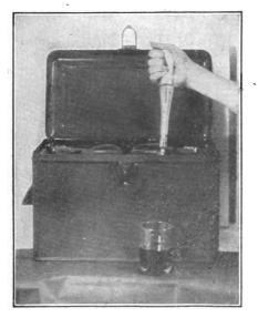
Fig. 25. Insert the Tube in Vent Hole in Center of Battery, and Squeeze the Hydrometer Bulb Until the Cell Is Filled to the Proper Level
