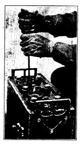
Fig. 107. Digging Compound from around Wells with Hot Screw Driver \*
