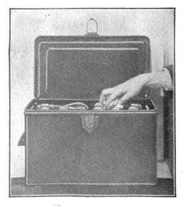
Fig. 27. Replace the Screw Plugs and Wipe Dirt and Moisture from Top of Battery
