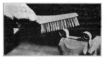
Fig. 156. Cleaning Connector Before Burning In
