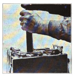
Fig. 171. Pressing Down Hot Top Connector Into No. 4 Compound. Willard Type S Battery
