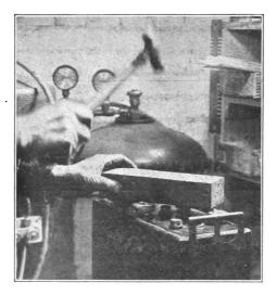
Fig. 157. Leveling Top Connectors Before Burning In
