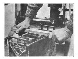
Fig. 148. Pressing Down Top Covers to Make Them Level with Top of Case
