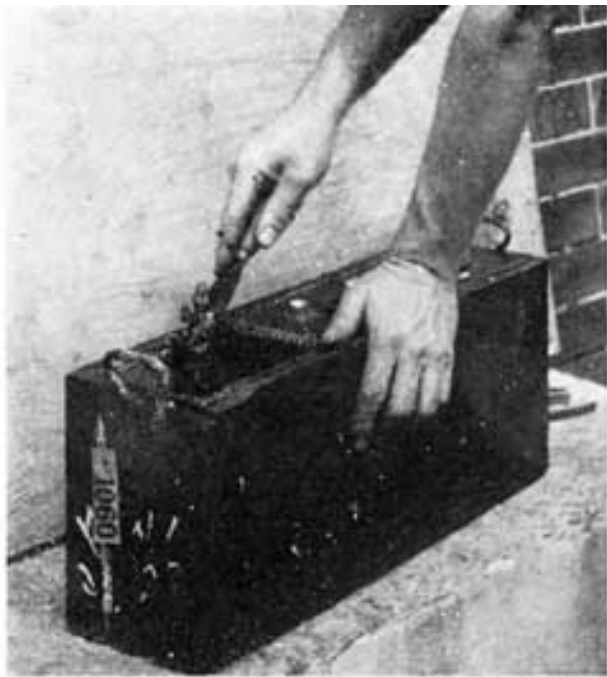
Fig. 200. Removing Compound from Top of Jar
