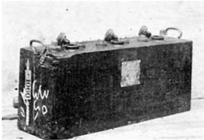
Fig. 195. Battery Ready for Steaming
