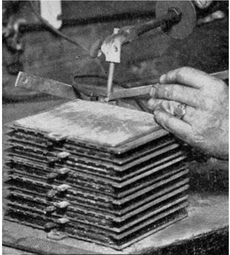
Fig. 322. Burning on Outside Negative Plate. Delco-Light Cell
