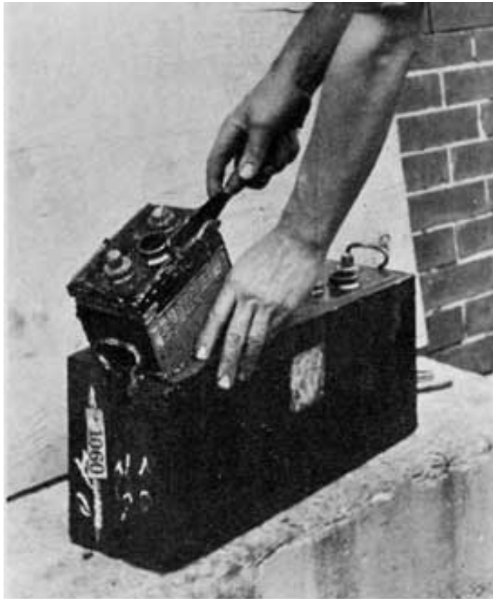
Fig. 198. Removing Compound from Cover
